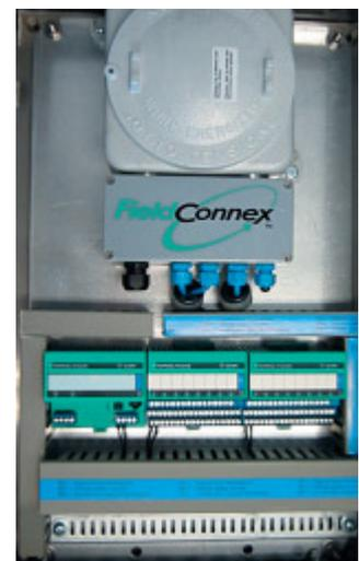
Figure 19: „Mini-RIO“ for installation in zone 1.
