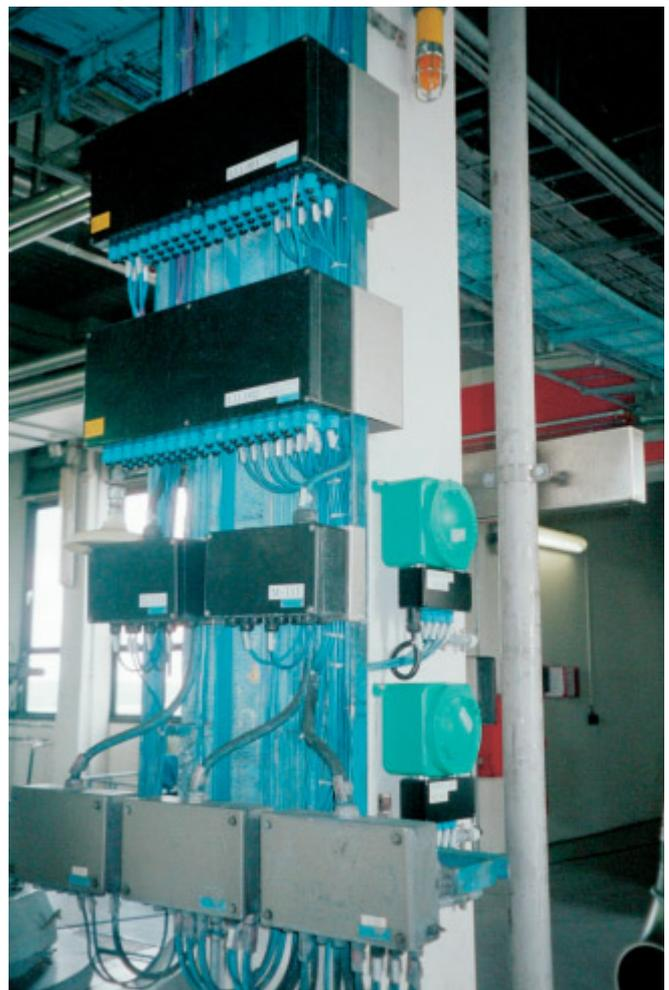
Figure 13: RIO system in central arrangement.
