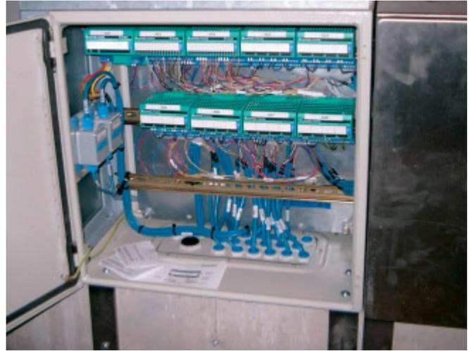
Figure 8: IS-RPI in the switch cabinet.
