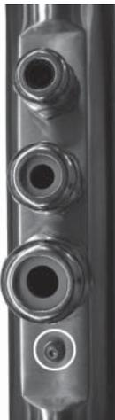
Figure 3.1: Ground connection at pedestal/wall arm
