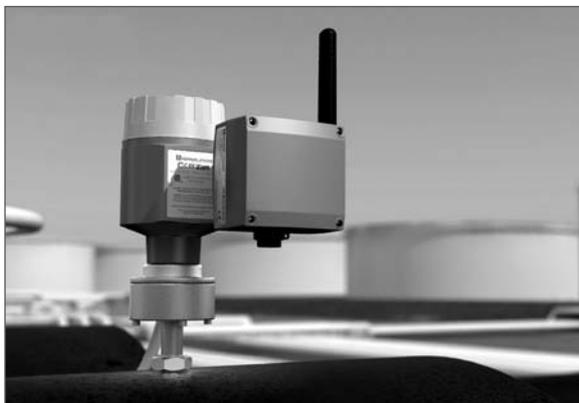
**Fig. 6: Wireless Corrosion Monitoring with *WirelessHART* Adapter**
