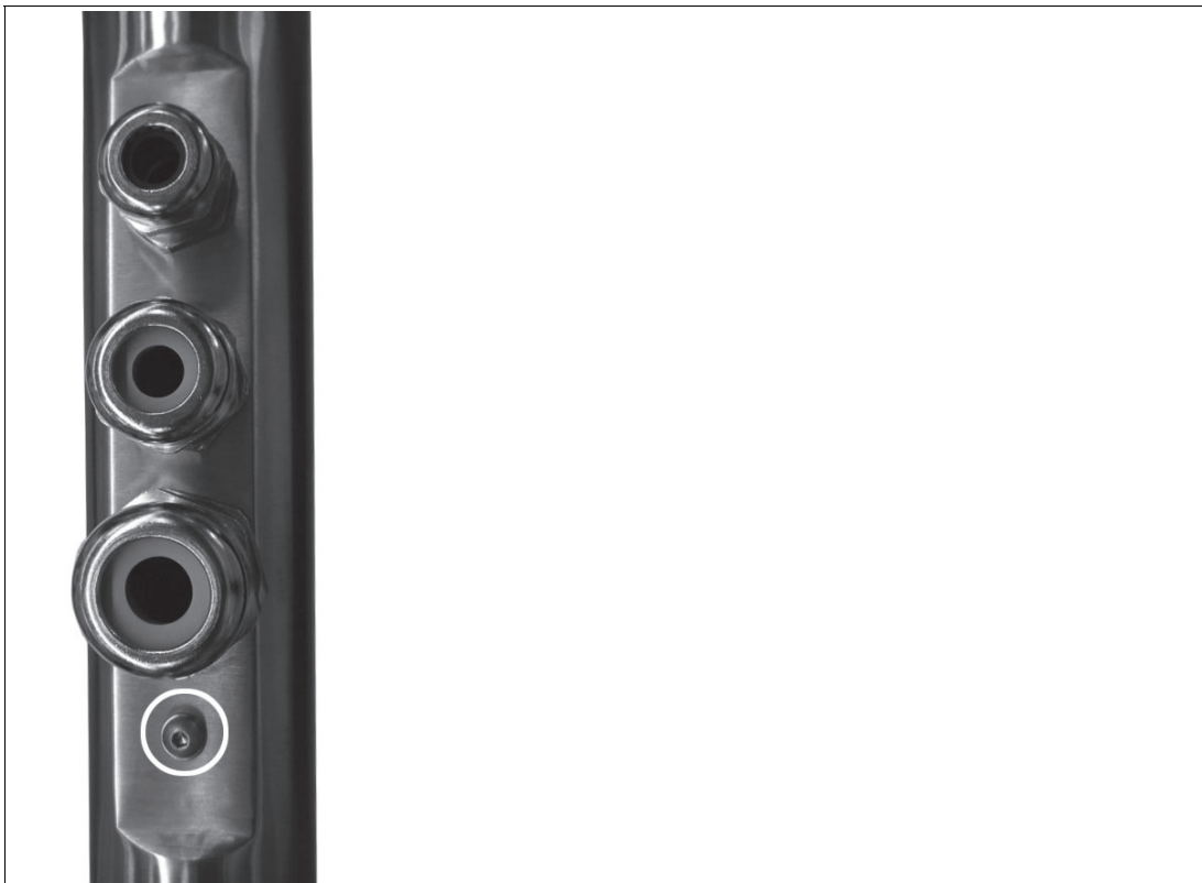
Figure 3.2 Ground connection at pedestal
