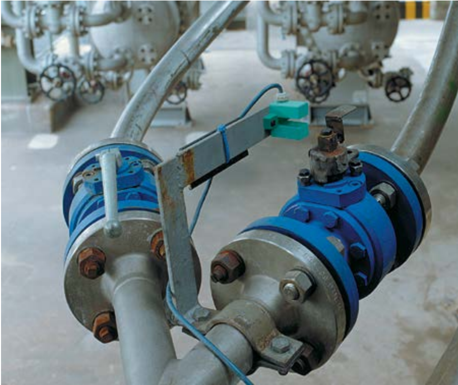
Figure 7. Valve status request with an Ex i sensor
