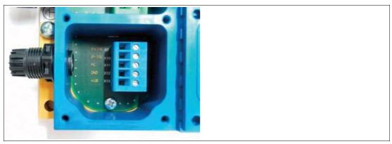
Figure 4.14 Intrinsically safe terminal compartment of the supply module after removing the connector connection cores
